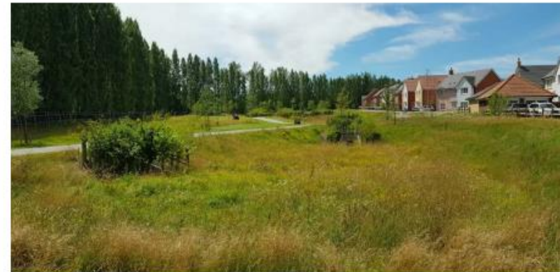
ATTENUATION BASIN (DAVENTRY) - AFTER ESTABLISHMENT OF LANDSCAPE
